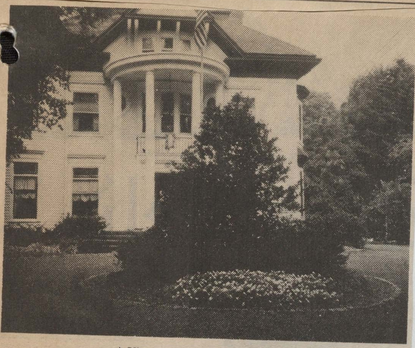
A Victorian house on the tour
